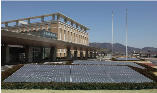
Figure 22: Solar energy panels Source: Nikken Sekkei Archits. & Engrs
