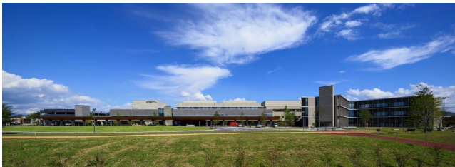
Figure 12: Overall view of the building showing patient ward and therapy wings standing side-by side
