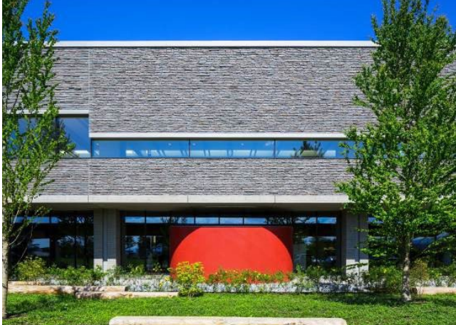
Figure 16: Façade incorporating locally produced Teppeseiki stone
