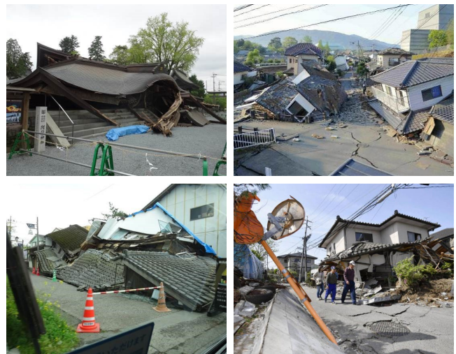
Figure 10: Damage from the Kumamoto Earthquake
