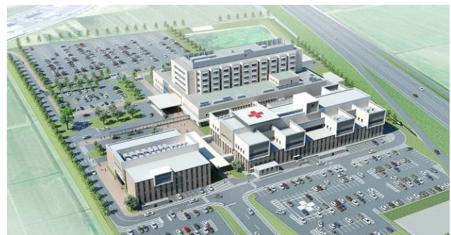
Overall view of the facility with new extensions
