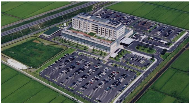
Figure 2: Hospital before disaster At the time of designing, the site was set aside 3 m in consideration of the history of the past damage, so it escaped flood damage.
