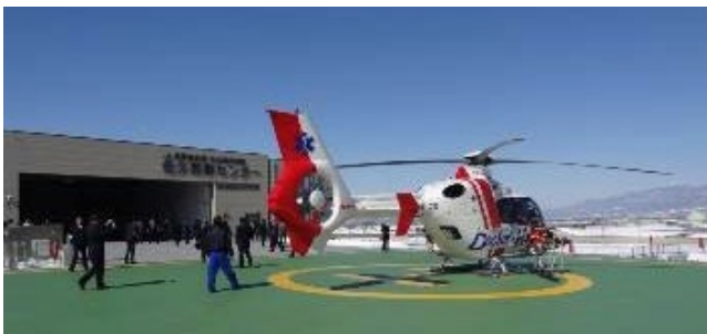
Heliport and helicopter ambulance hanger
