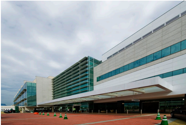
Unimed Hospital Main Entrance
